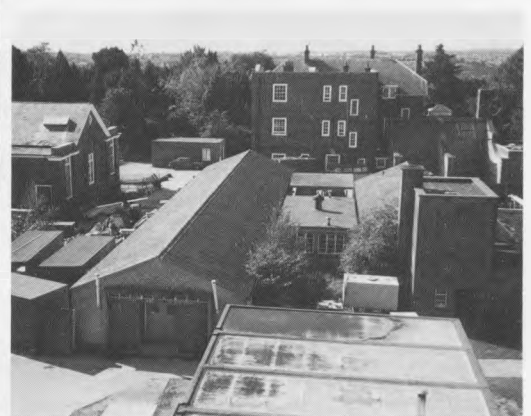
Above: The area to be demolished after completion of the VI Form/canteen/sports complex.
